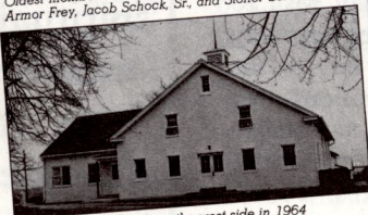
An addition was built on the west side in 1964
