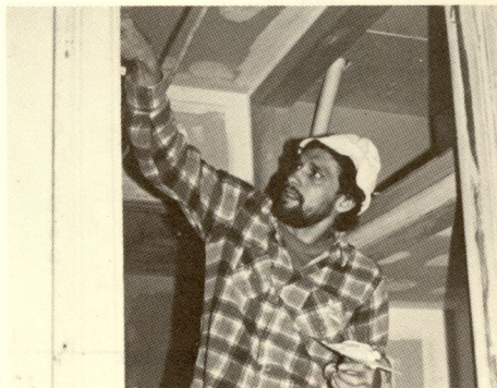
Renovating homes, Washington, D.C.
