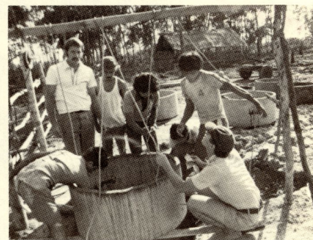
Well construction, Indonesia
