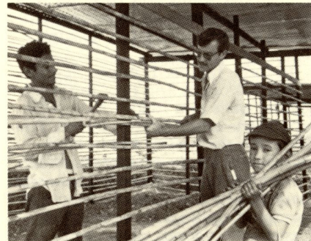
Housing construction, El Salvador
