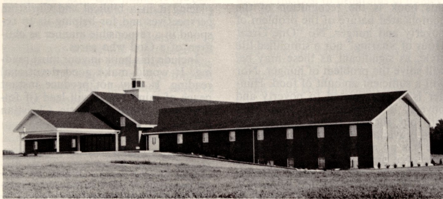
A view of the newly remodeled and enlarged Cross Roads Church.
