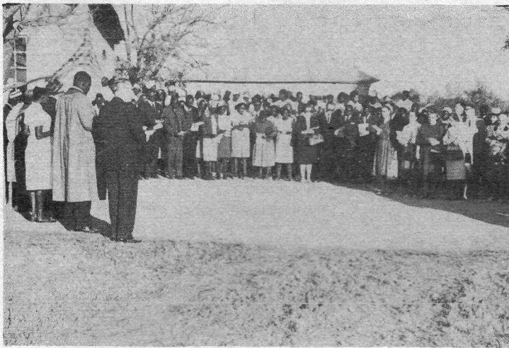
A portion of the group attending the Groundbreaking Ceremony for the pediatrics ward and tuberculosis ward at the Mtshabezi Hospital. The pediatrics ward will be located to the left rear. The tuberculosis ward will be in the foreground. The string marking proposed front veranda.
