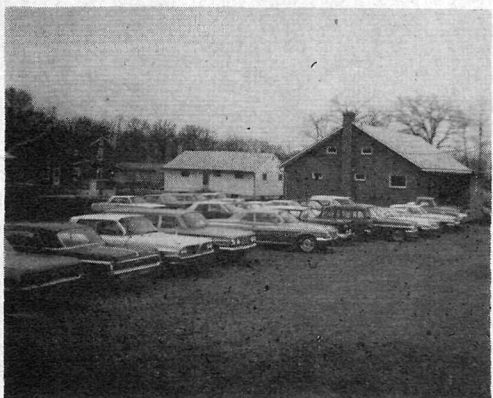
View of parking lot and rear of the church.
