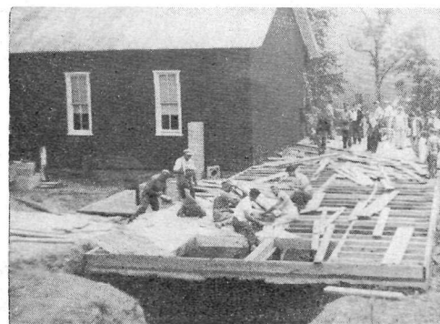
Addition being built to the Sherman's Valley church.
