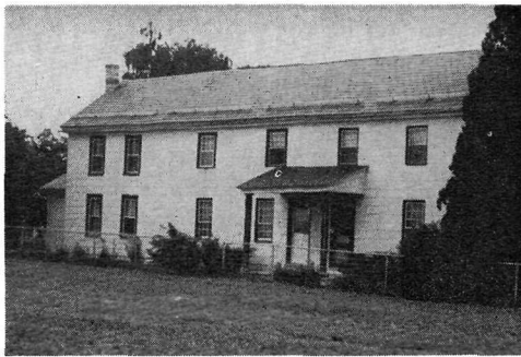
Engle House where services were held. House is constructed for rooms to be joined together, making something of an audience room. A small shelf still remains where the song-books were kept.
