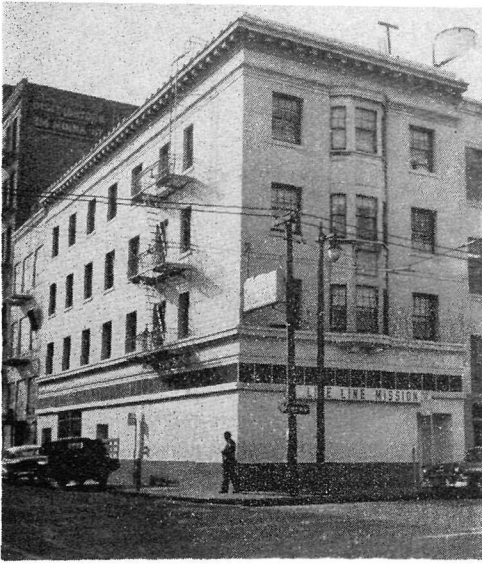
The completely renovated Alpine Hotel, now the Life Line Mission, holds out a ray of hope for the lost souls of San Francisco's Skid Row. During the last year, 337 gospel services were held; 51,244 free meals were served.
