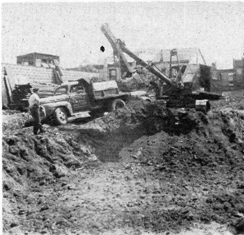
Excavation for the new church at Philadelphia, Penna.
