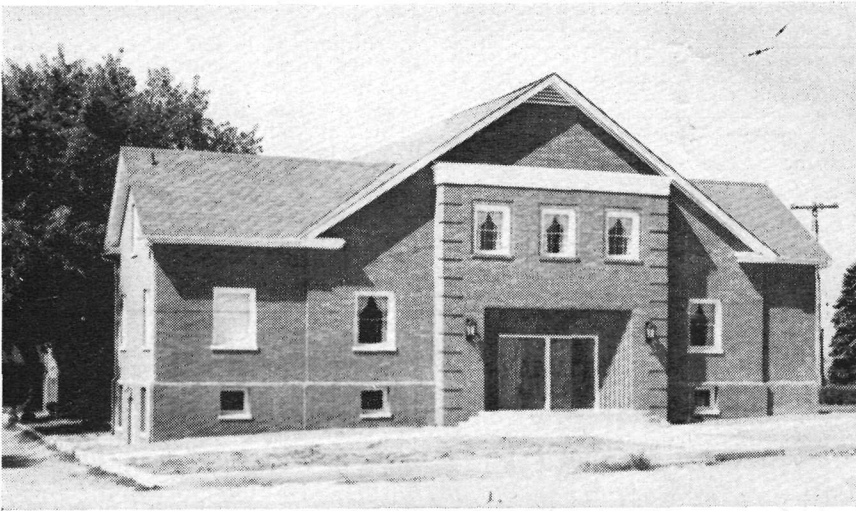
Front view of the remodeled Cross Roads Church
