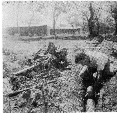
Dr. Engle laying sewage pipe for the drainage system.
