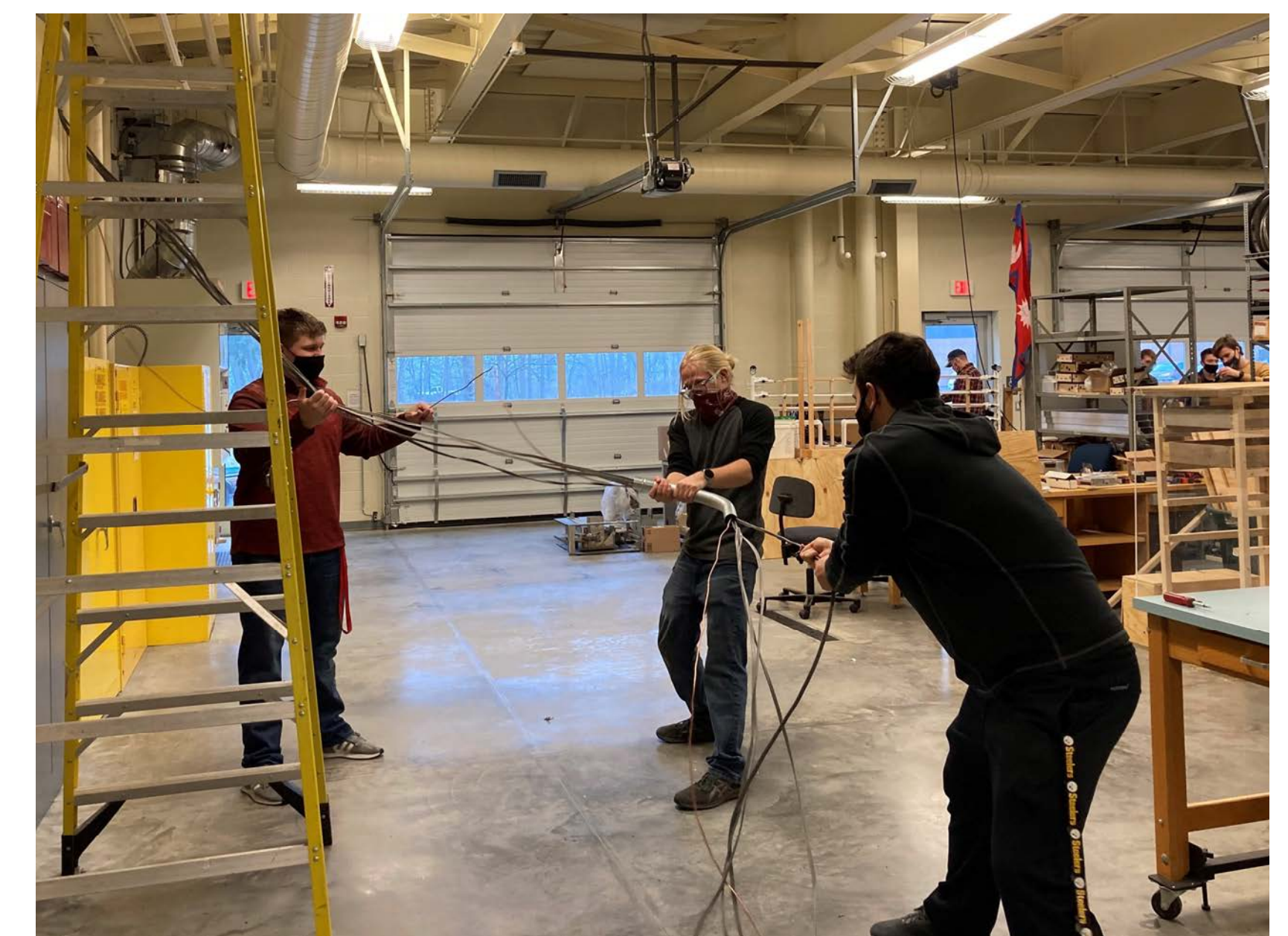
Figure 4: Pulling wire through conduit
