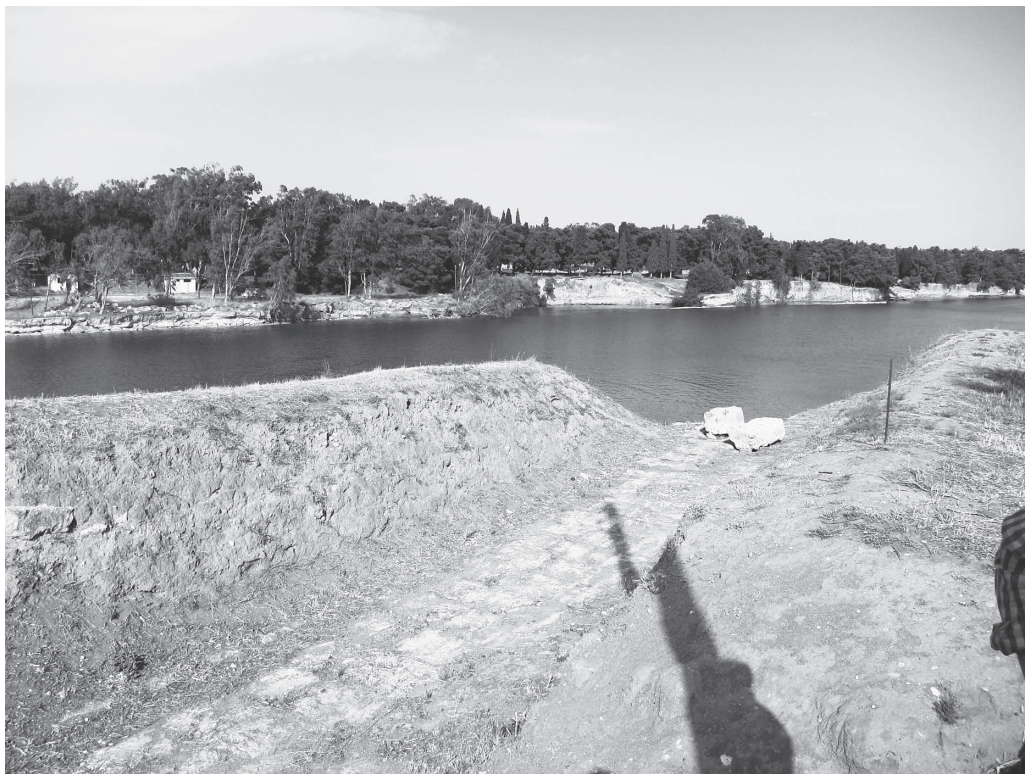
Fig. 8. Sector G of the portage road in 2011, where the modern canal bisects it. Some 10 m or more of the road has fallen into the canal through neglect.
