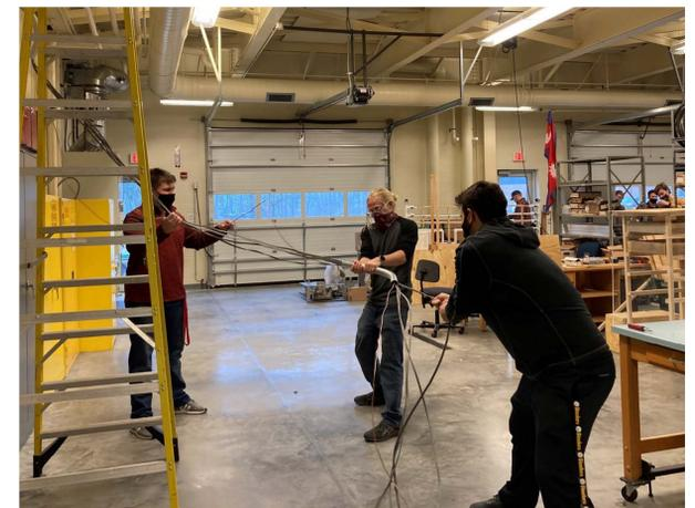
Figure 4: Pulling wire through conduit
